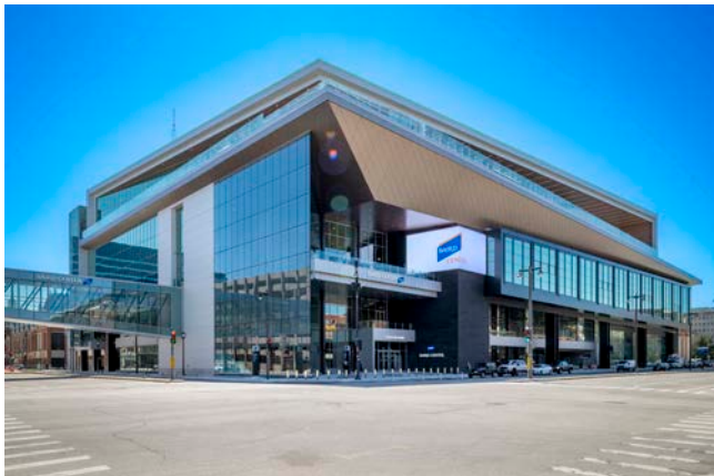
Baird Center, Milwaukee
